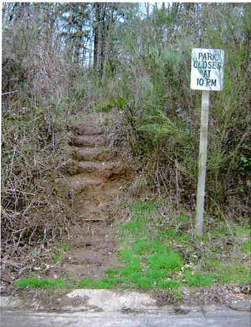
Entrance needs work
